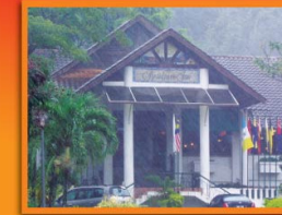
Residence Inn, Cherating
